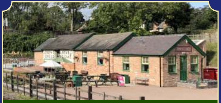
ELLIS TEA ROOM EXTENSION & REFURBISHMENT
