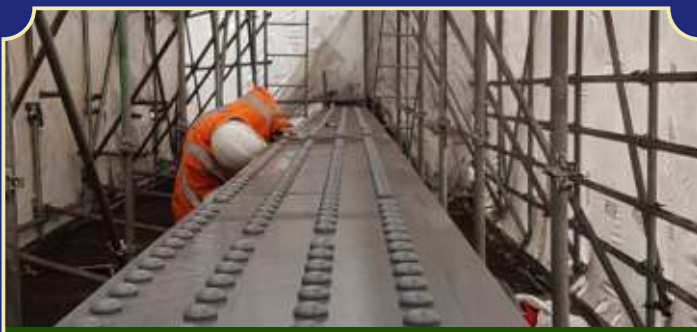
CANAL BRIDGE - REPAIRED AND RESTORED
